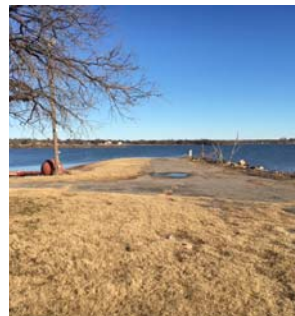
Boat ramp cleanup in progress
