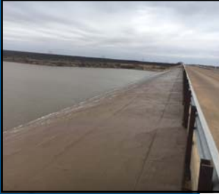
Water going over the spillway, March 2017
